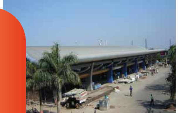
Pune International Airport, India Product Used: Kalzip Standing Seam System
