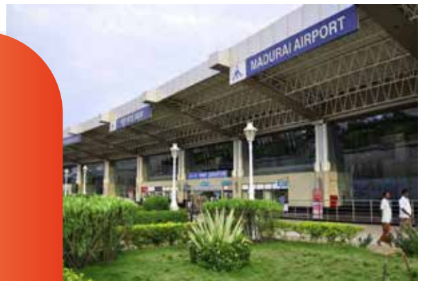
Madurai Airport, India Product Used: Kalzip Standing Seam System
