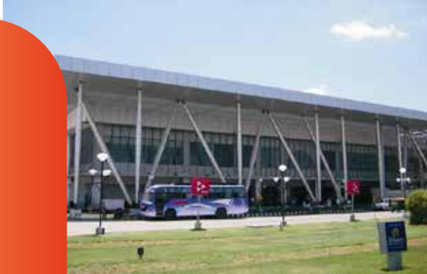
SVP International Airport, Ahmedabad, India Product Used: Kalzip Standing Seam System
