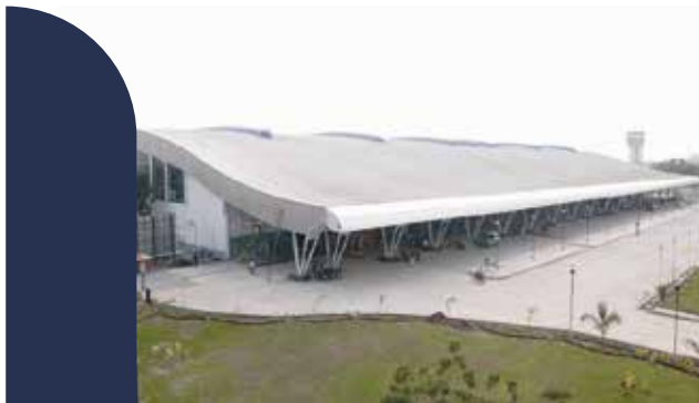
Aurangabad Airport, India Product Used: Kalzip Standing Seam System
