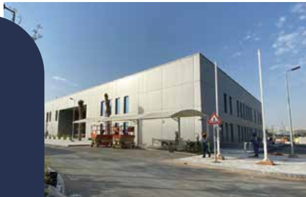
EXPO Operation Centre EXPO 2020 Dubai
