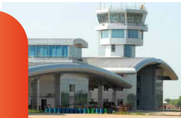
Gondia Airport Hanger, India
