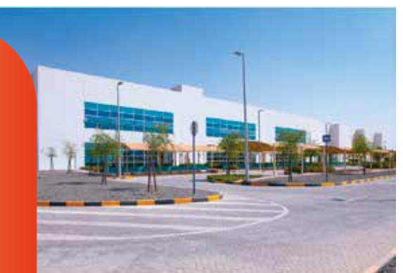
Khazna Data Center, Abudhabi, UAE
